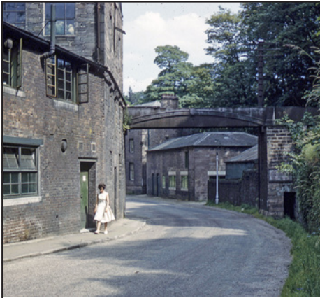
The cast-iron aqueduct that carried the water of Cromford Sough across the road to Arkwright's Mill, photographed in the early 1960s, when the buildings were still in use by the colour works.
