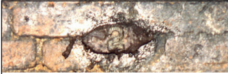
One of the chain markers indicating the distance into the tunnel.
