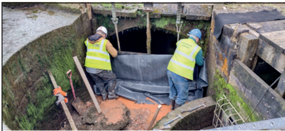
Fitting the synthetic rubber sheet.
