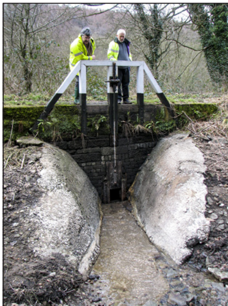
The sluice opposite Aqueduct Cottage is one of those Frank Bark describes for draining sections of canal.
