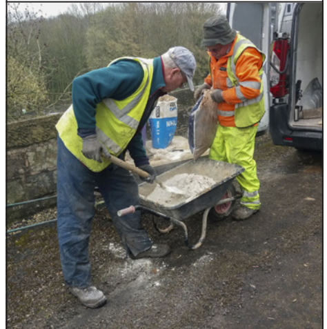
Mixing the lime mortar.
