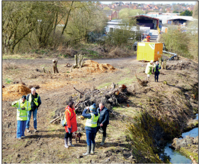
FCC members show funding consultants from Marsha Miles around the Beggarlee site, with the new crew cabin in the background.
