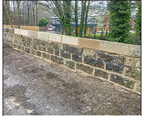
The completed parapet wall at Sawmills.
